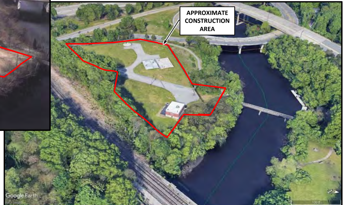
Shaft 5/5A, Weston – Post Construction
