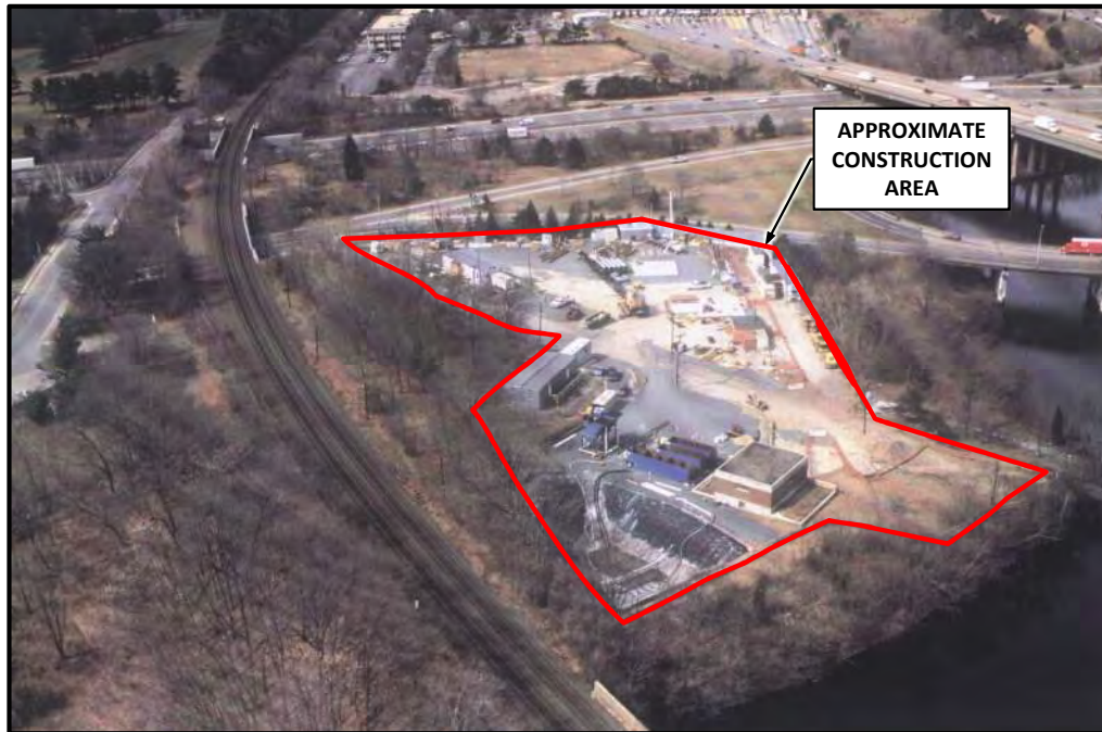
MWWST Shaft 5/5A, Weston – During Construction
