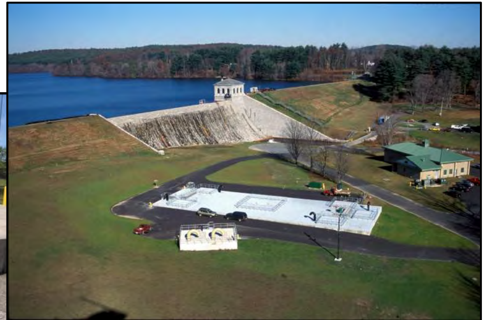
MWWST Shaft E, Southborough
